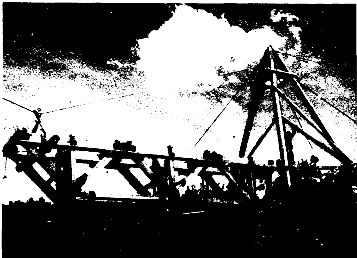
Launching a pair of trusses during the construction of a low-cost modular prefabricated wooden bridge (Honduras)
