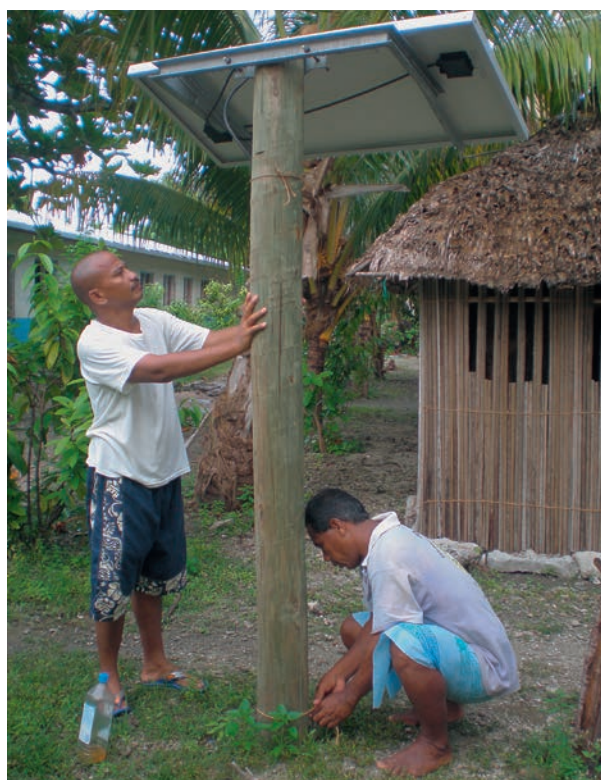
Installation of photovoltaic units in the Pacific Island region.
