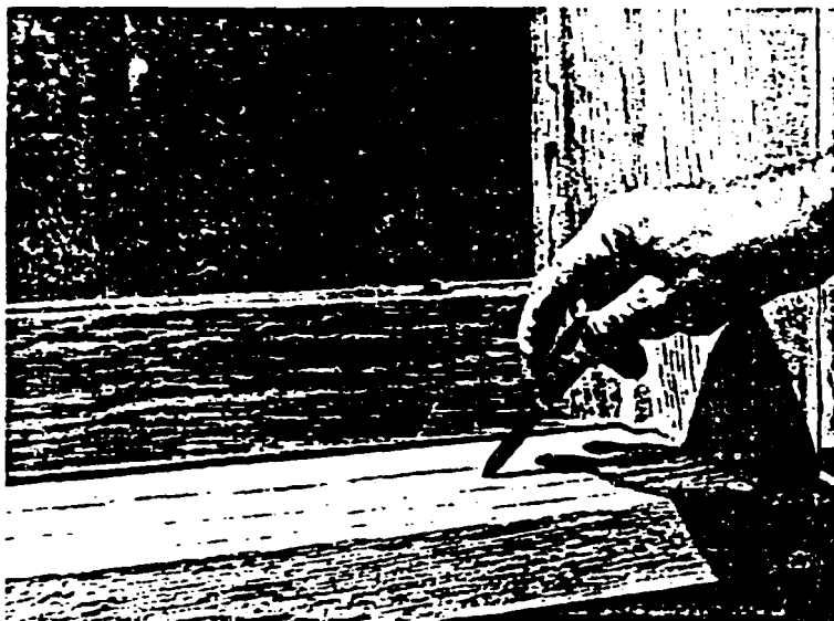
Figure 4.—Closeup view of water-repellent-protected window unit and frame after 20 years' exposure. Firm wood resists penetration by the knife blade. M 145 288-16
