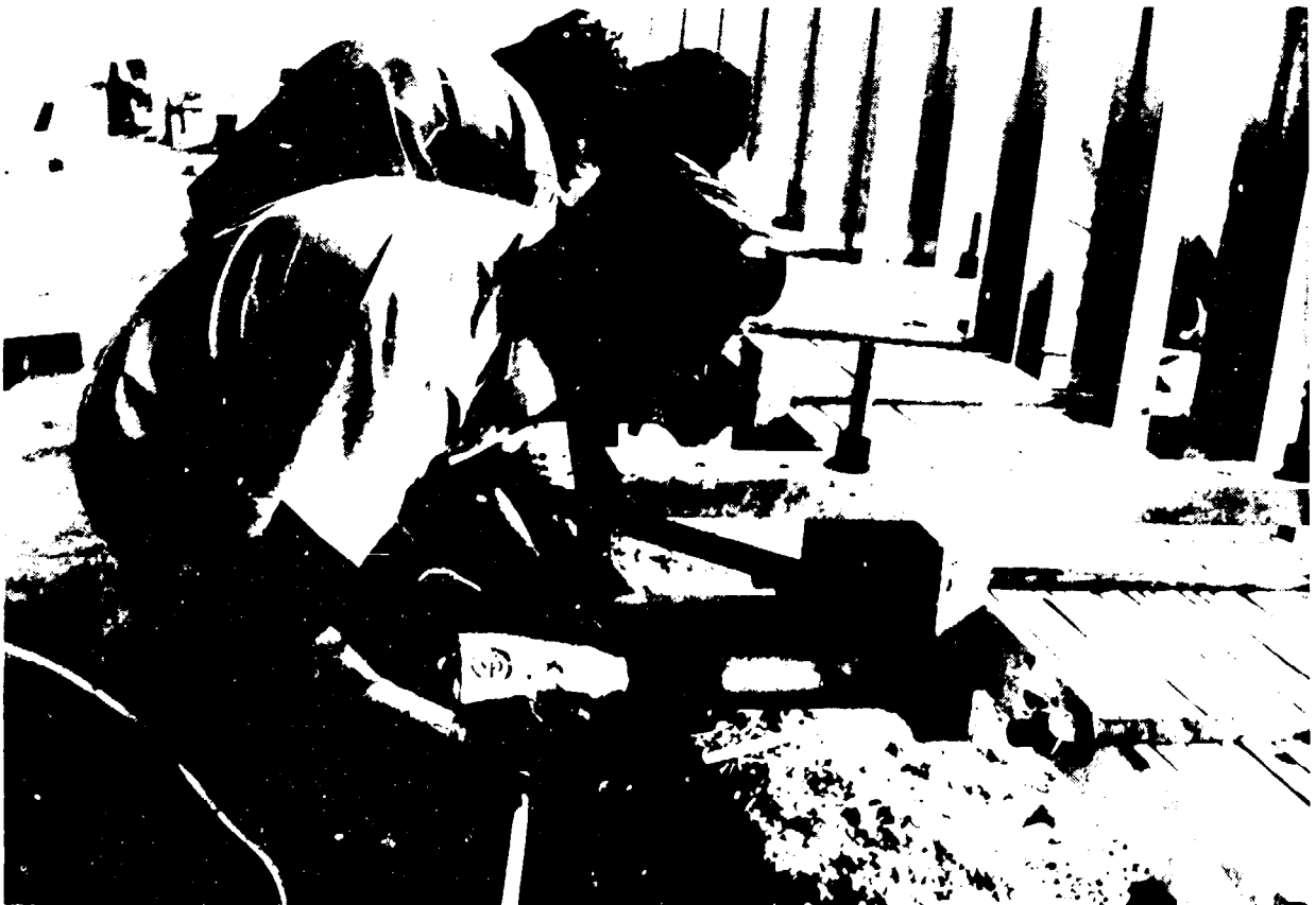
(b) Pneumatic impact wrench with adapted deep socket in use
