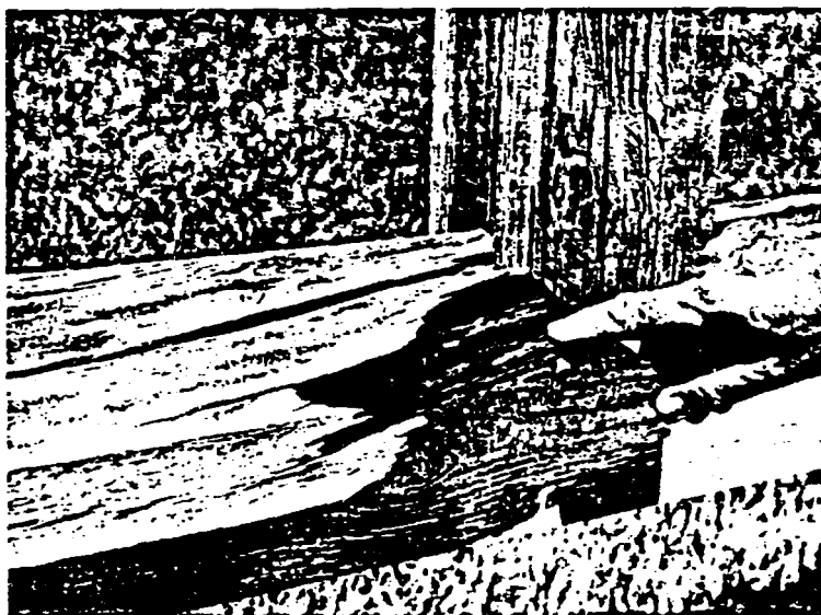
Figure 5.—Closeup view of decayed untreated window unit frame. Window unit fell apart after 6 years' exposure. M 145 288-8
