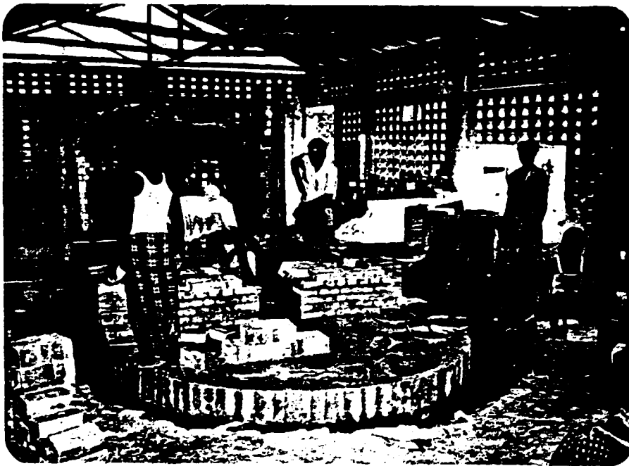
Construction work on throat and tank
