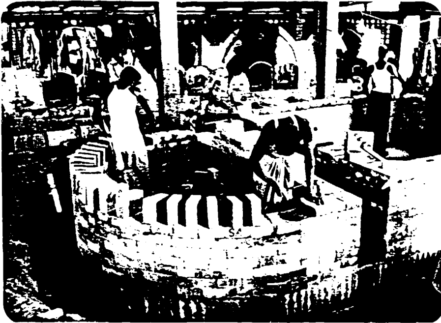
Construction work on refiner and tank of a glass melt furnace
