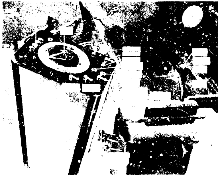
Fig. 27: Typical older type control panel.
