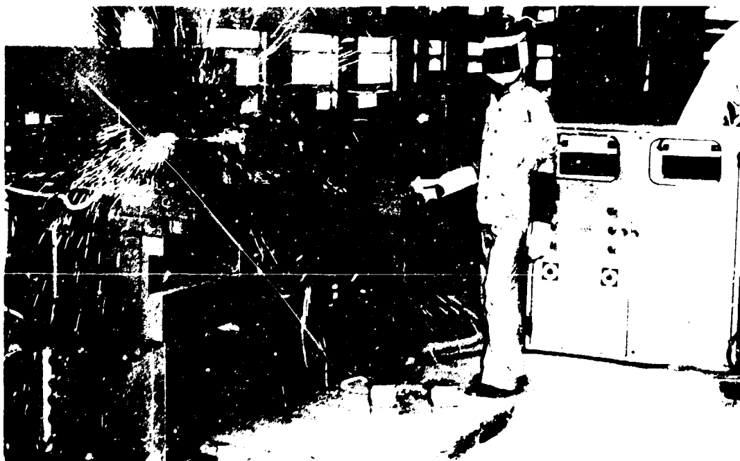
Flash butt-welding of tubes in progress at Welding Research Institute, Tiruchirapalli, India
