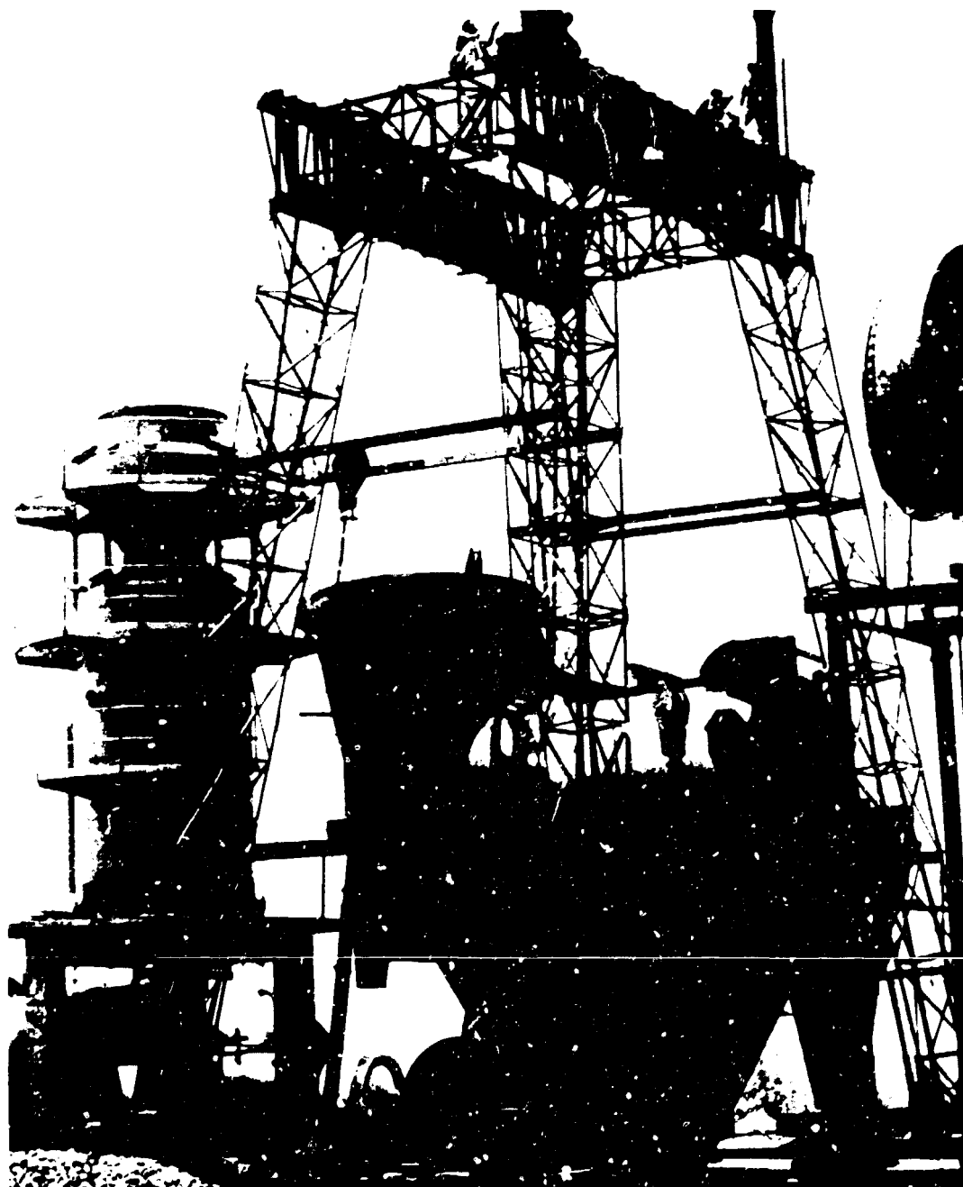
Installation of after-burner and stack of the rotary kiln for the demonstration sponge-iron plant, Andhra Pradesh, India
