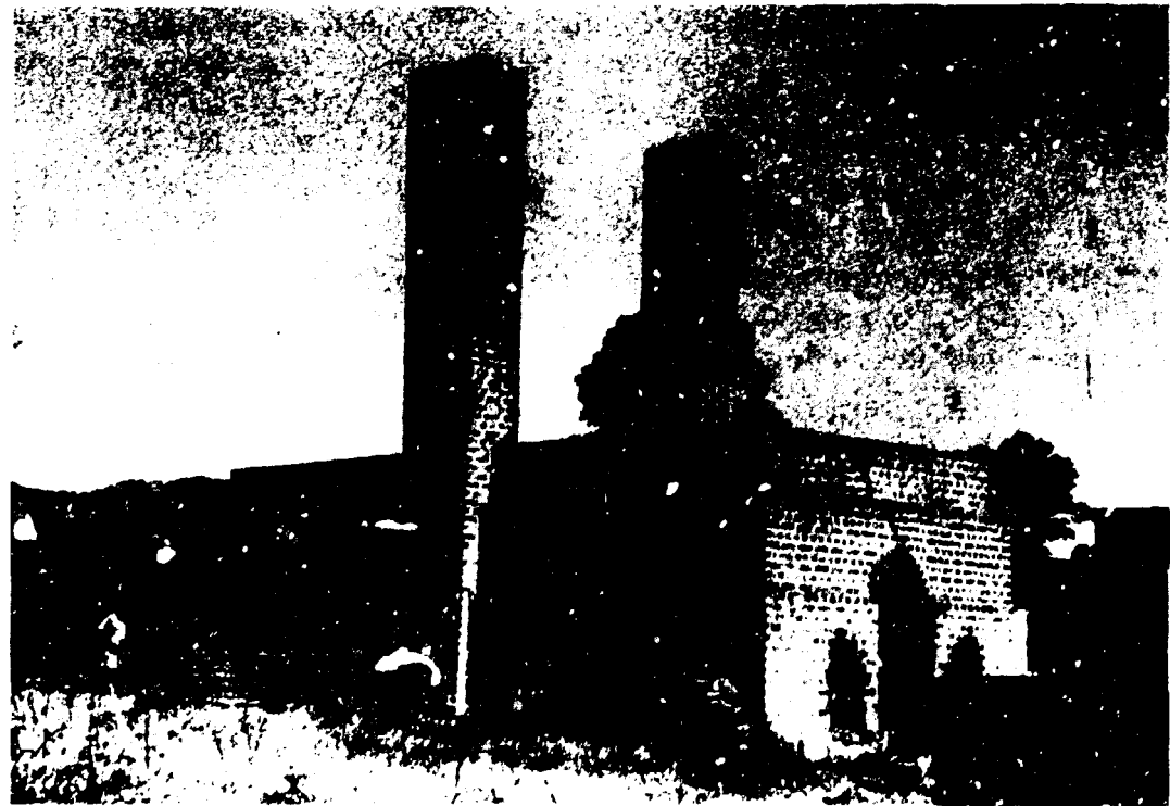
A demonstration brick kiln built in Blantyre, Malawi
