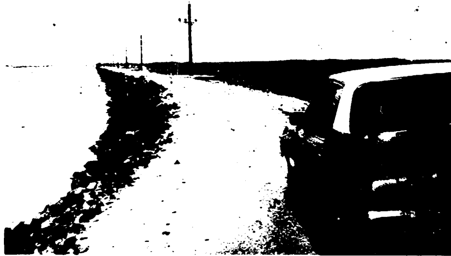
Fig. 6.4 Internal embankments lined with boulders
