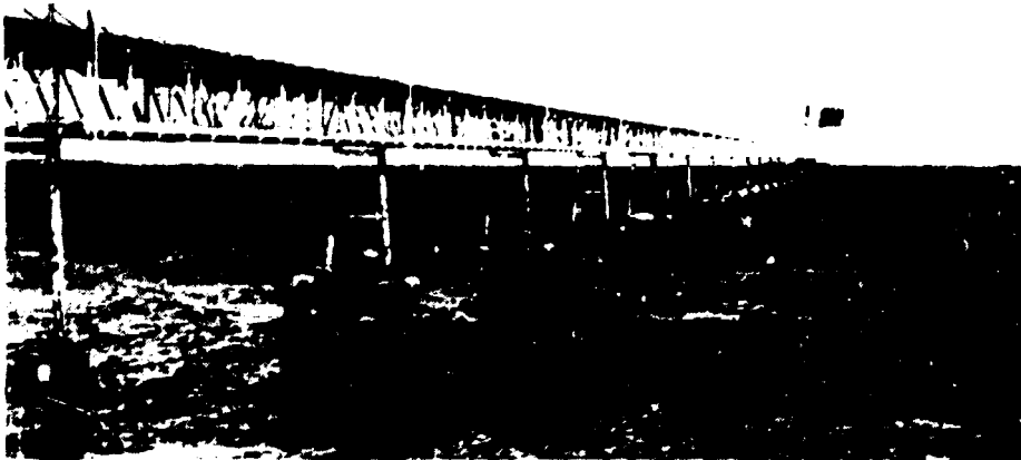
Fig. 6.13 Jetty for direct loading of salt into ships
