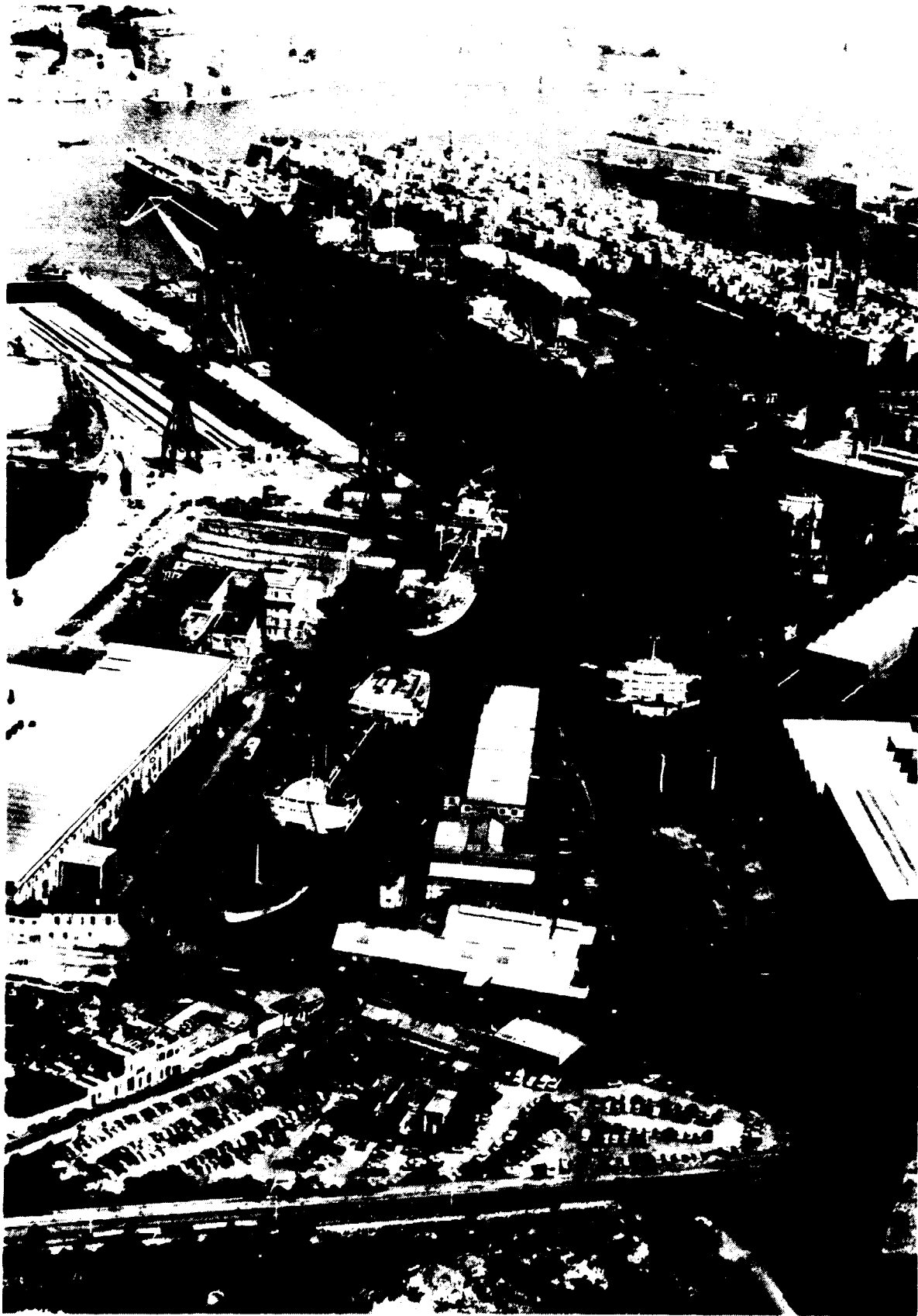
General view of Malta Drydocks showing Nos. 4, 5 & 6 docks also the partially completed No. 7 dock.
