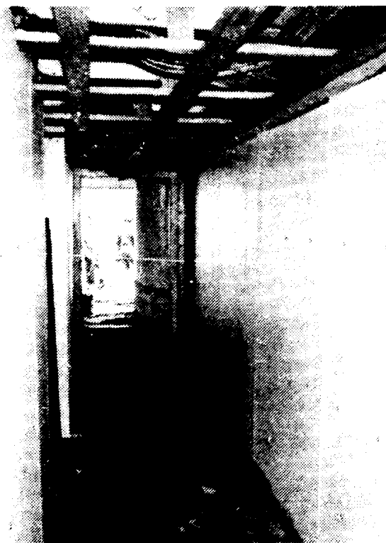
New alleyway in accommodation area under construction.
