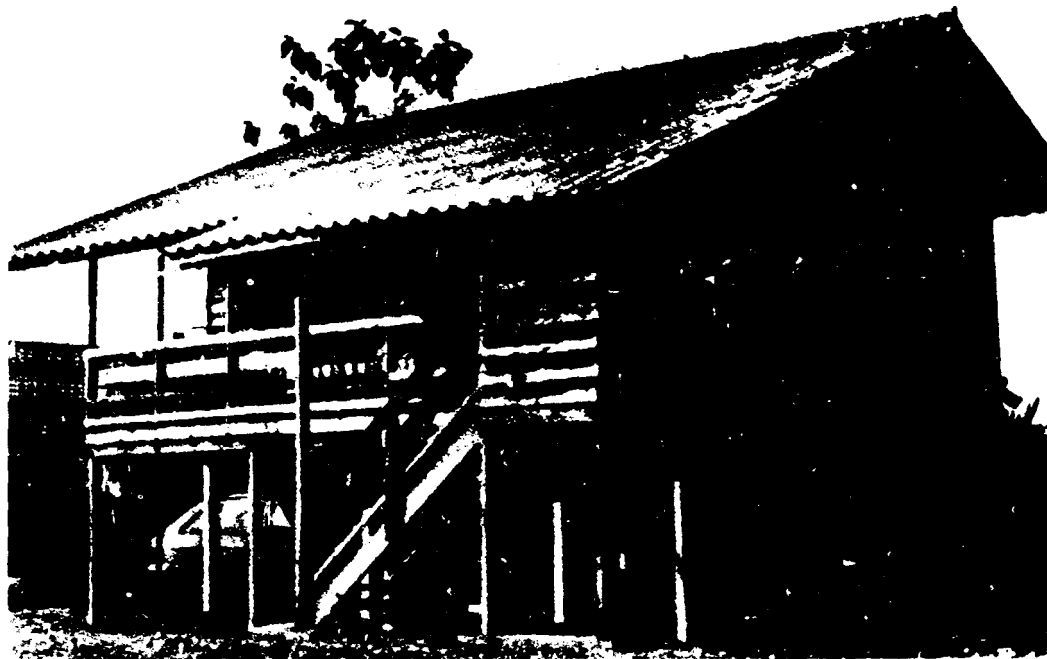
School in the Lao People's Democratic Republic using a low-cost modular prefabricated building system
