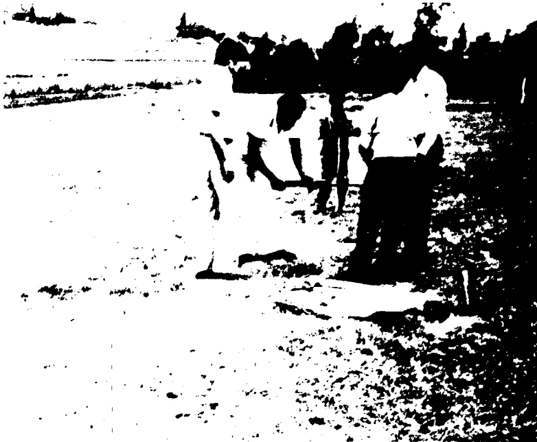
Checking the Alemgena site for possible load bearing qualities.
