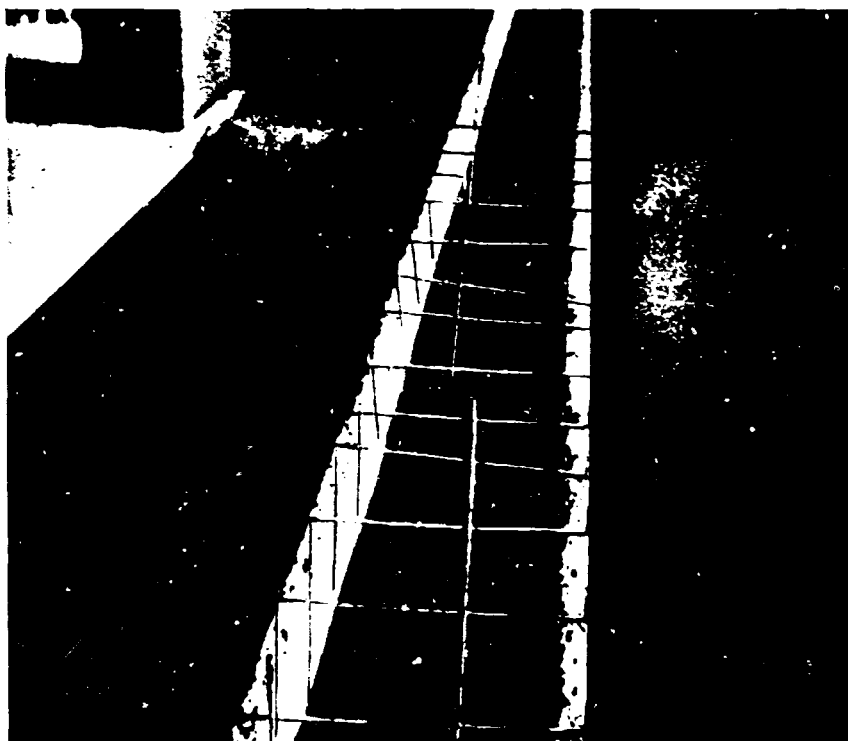
Fig. 57: Wood-wool cement board blocks with steel reinforcing rods.
