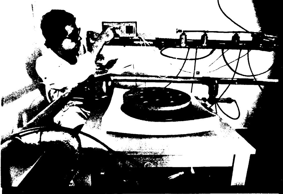
The table top is tested with water, coffee, alcohol, acetone (desks), grease, heat, and scratching.
