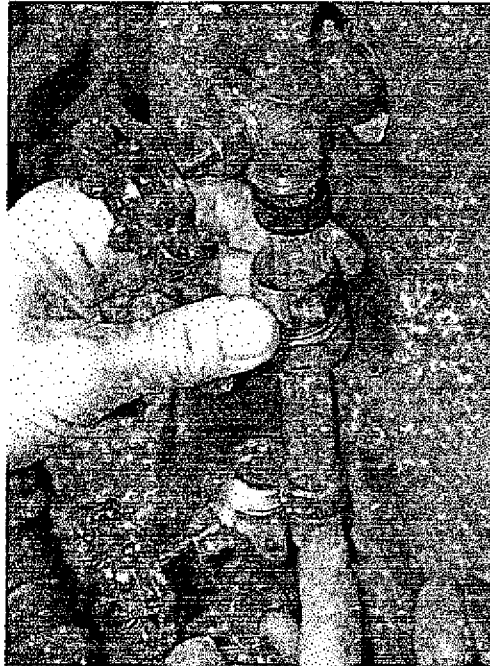
Inserting sight glass into valve assemblies
