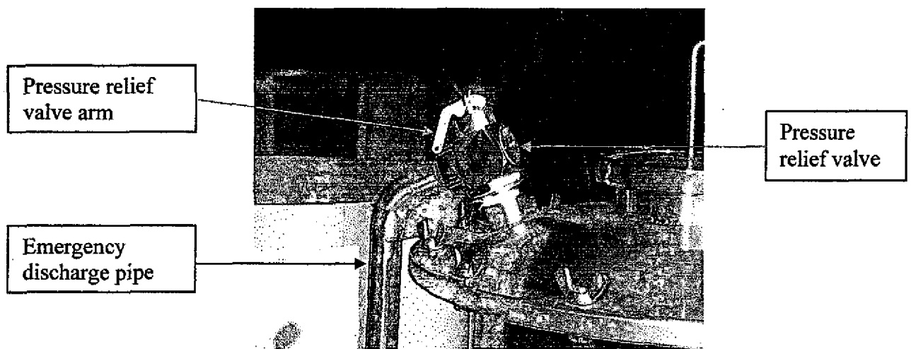
Pressure relief valve assembly
