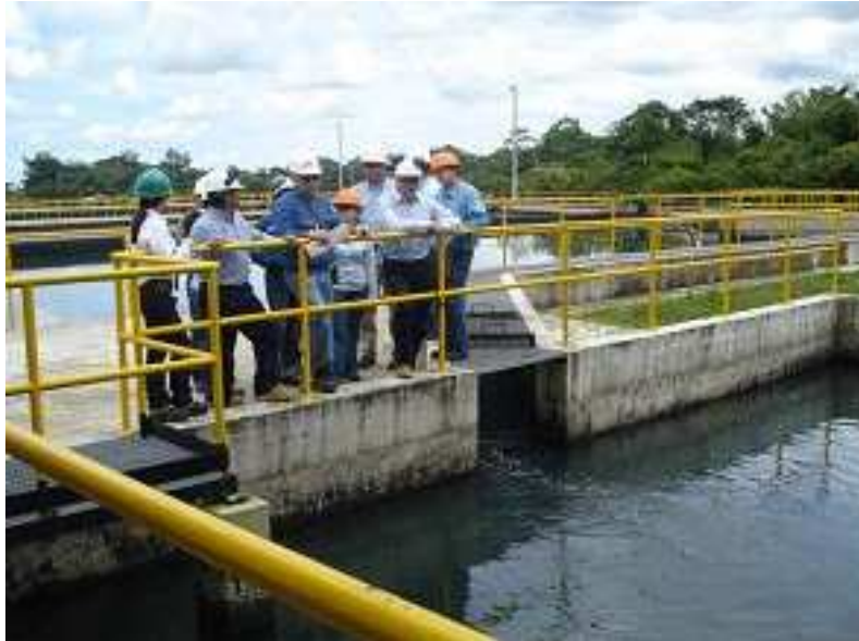
Process: Water clarification and crude dehydration in Castilla field–Villavicencio Colombia-
