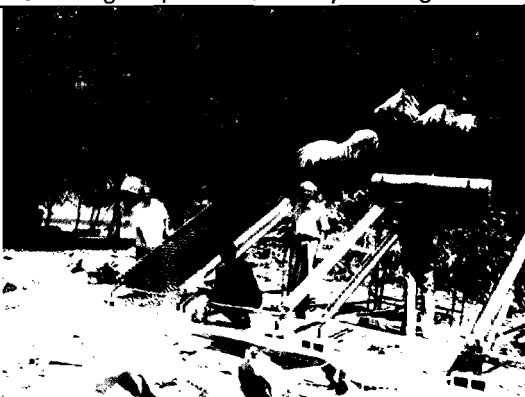
Shifted for more sunlights , work in progress
