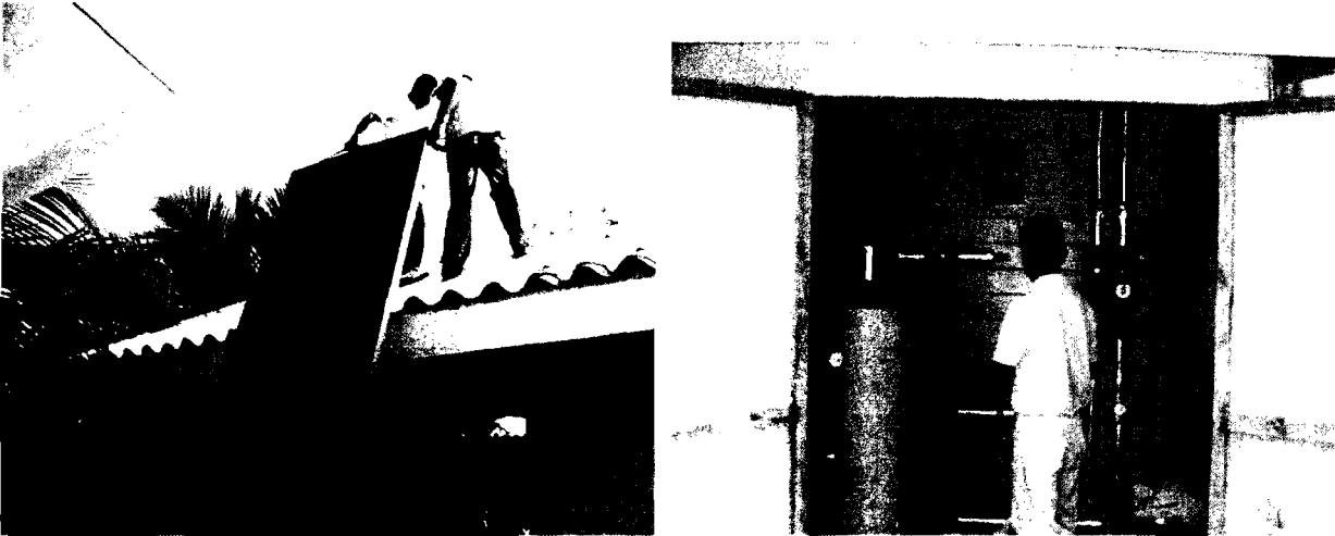
Figure 11: Installation work at the hotel Vistamar - System 1
