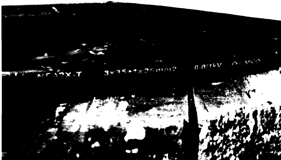
Picture 41 : One of cable type which is used for transmission lines
