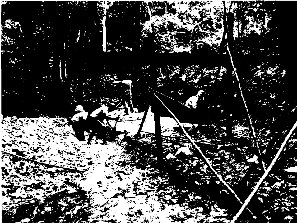
Picture 7 : Excavation work
