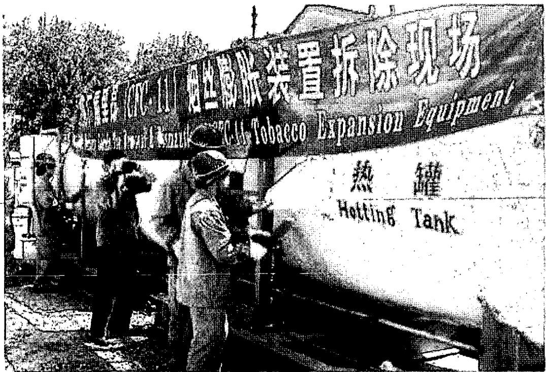
The CFC-11 equipment locale for dismantle
