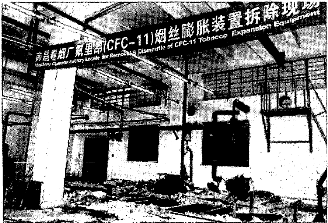
Dismantle Scene (The CFC-11 equipment had been dismantled)
