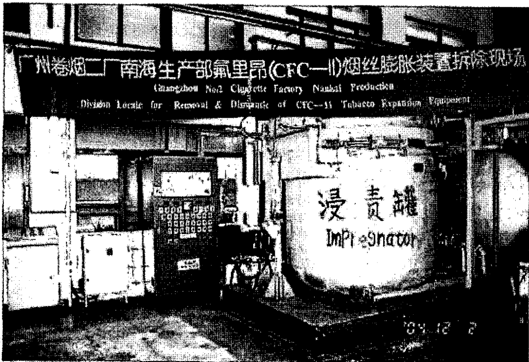
The CFC-11 equipment locale for dismantle
