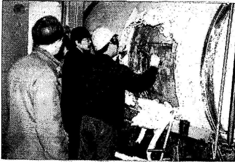
Dismantle Scene (The CFC-11 equipment was dismantling)
