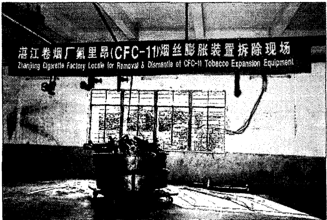
Dismantle Scene (The CFC-11 Equipment was dismantled )
