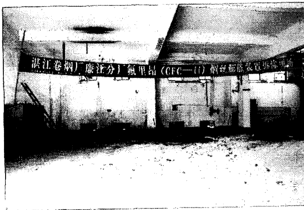
Dismantle Scene (The CFC-11 Equipment was dismantled )
