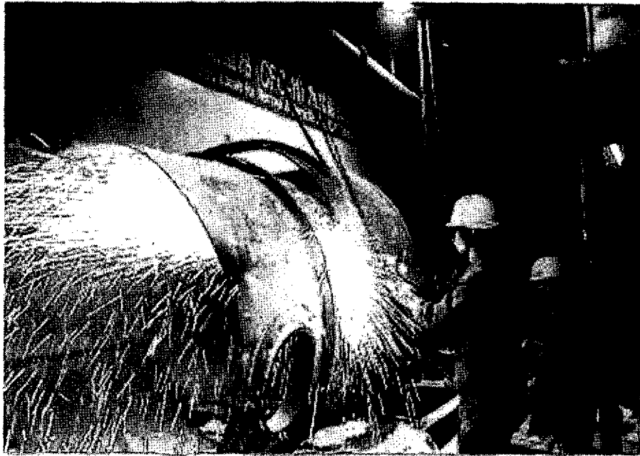
Dismantle Scene (The CFC-11 equipment was dismantling)
