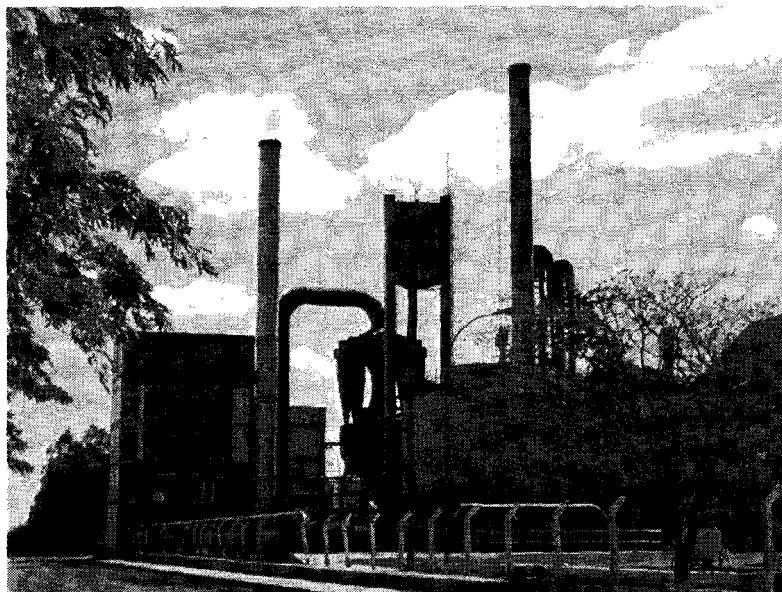
Figure 9-1 The CHP plant at CAMIL Itaqui [63].
