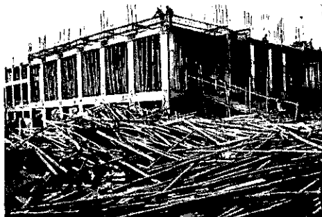
Bamboo used as scaffolding
