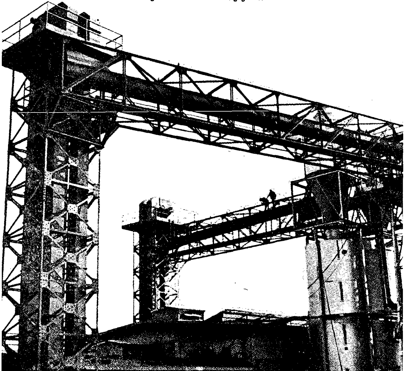
Figure 30. A wind-sifting grader
