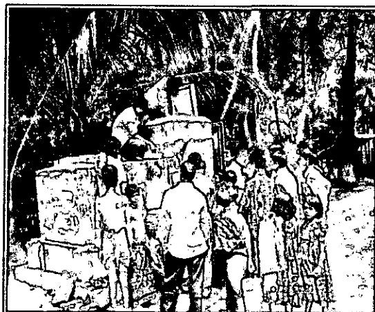
Maintenance & backwash of CBARU by the Users and UNIDO Arsenic Project personnel
