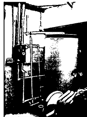
Figure 24: Collector area (left) and hot water storage tank 1000 litre (right)
