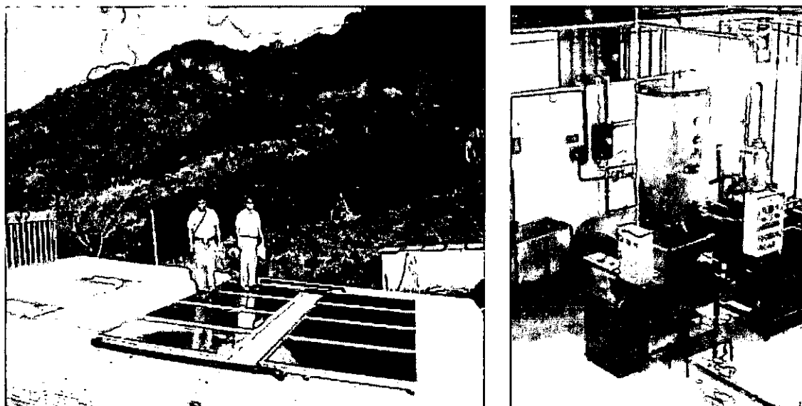
Figure 15: Installed solar thermal system at Lácteos Santa Martha
