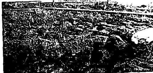
Fig 176- Root of the red mangrove used on the base of houses as barrier to sea upsurge
