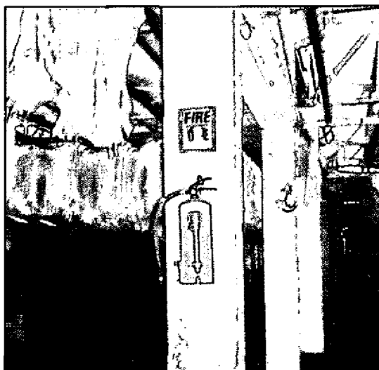
Keep fire fighting equipment ready in marked locations. (Photo: RePO-UNIDO)
