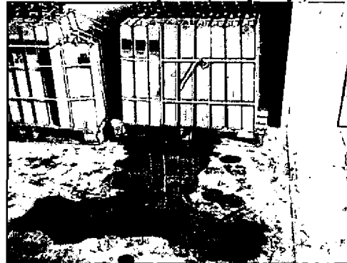
Picture 76: Bad Example II (no tip trays)
