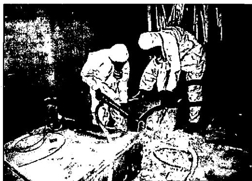
Picture 53: Sealing-off of a Contaminated Zone by Protective Tent with Compartments
