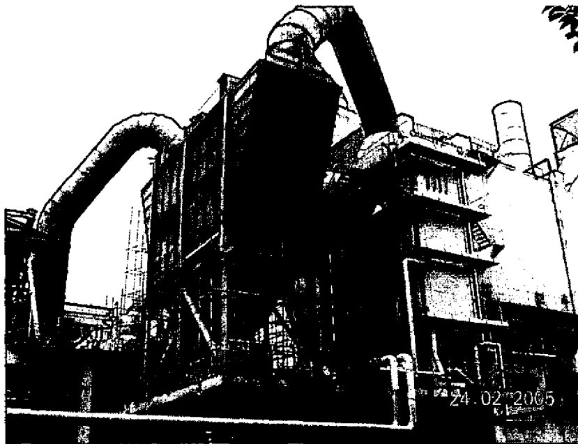
The Kiln Inlet Waste Heat Boiler
