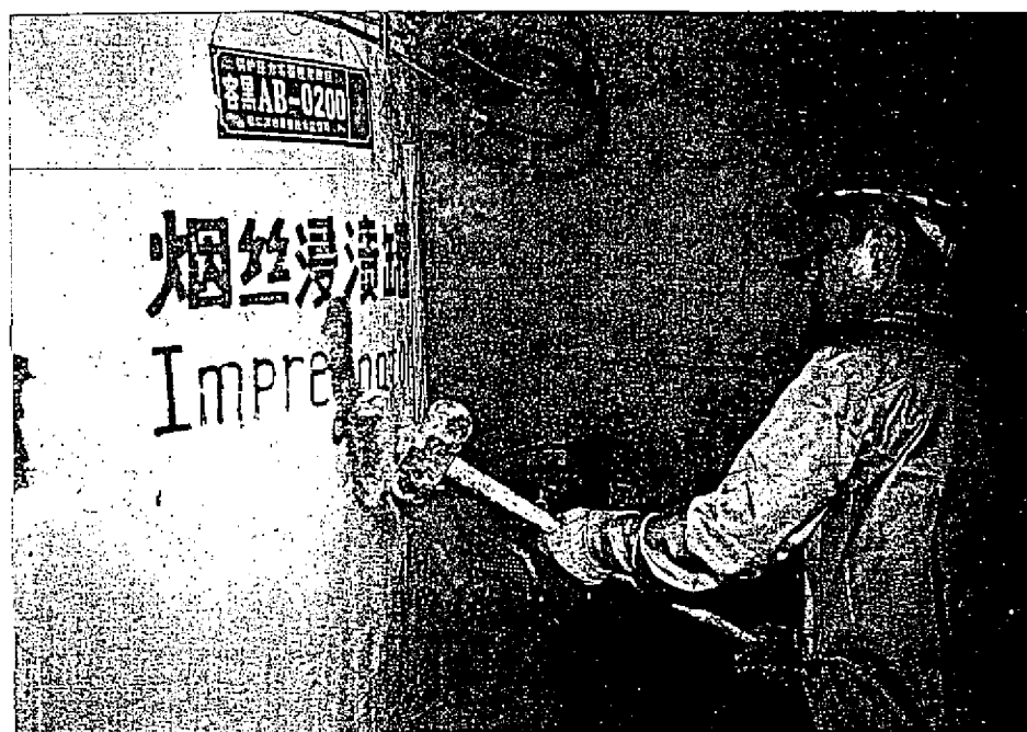
Dismantle Scene (The CFC-11 Equipment was dismantling)
