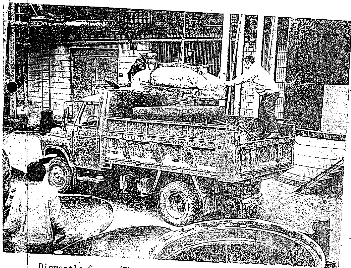
Dismantle Scene (The CFC-11 Equipment was dismantling )
