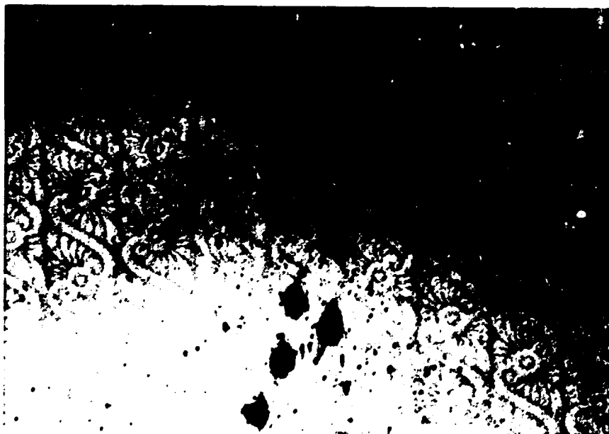
Figure VII. Stains from hot-air stenter exhaust pipe
