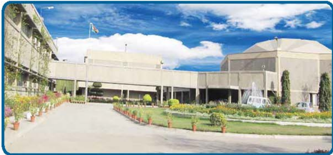
NCCBM Building, Ballabgarh, Faridabad, Haryana
