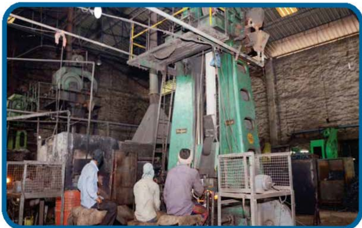
Forging press in Jalandhar Hand tools Cluster
