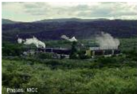
Figure I. The Olkaria I power station in Kenya
