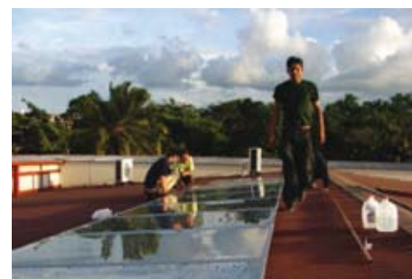
Installation of the solar thermal system at Hotel Mansión Teodolinda
