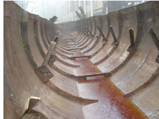
Emergency tank interior after cleaning (Source: Pure Earth)
