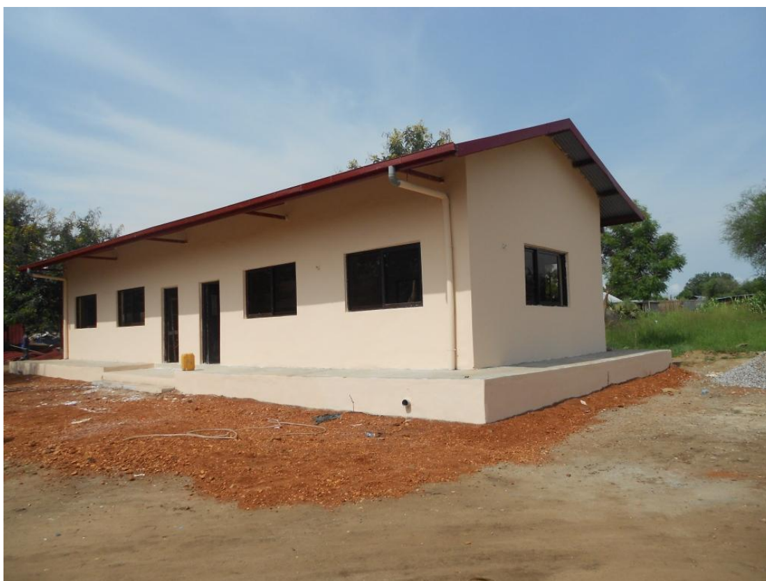
Picture: Training building completed as part of the building and Construction training in St Vincent
