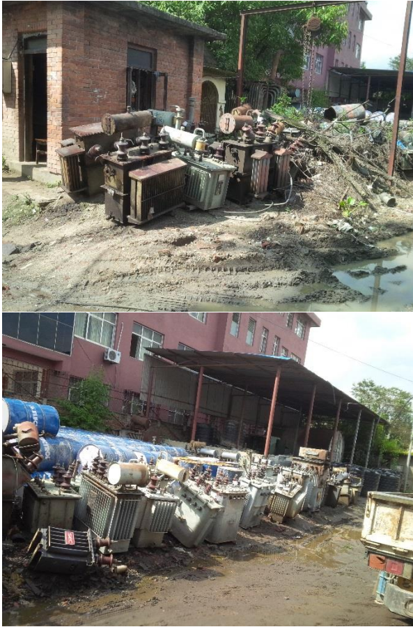
Figure 1: Old transformers stored in the open at NEA transformer workshop, Lainchaur
