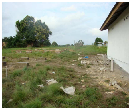
Figure 11 - Battery house at Harper with solar panel plinths behind
