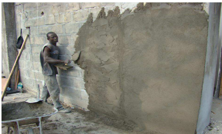
Figure 13 - On-the-job training at the RSTI construction site
