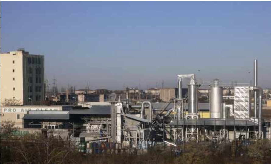
Figure 3: The facilities of PRO AIR CLEAN S. A.
