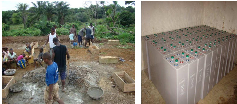
Figure 17a - Pujehun Growth Centre 11 kW PV system in construction
