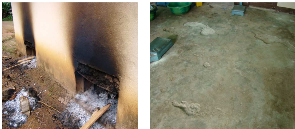
Figure 18 - Construction rehabilitation required at Pujehun GC
