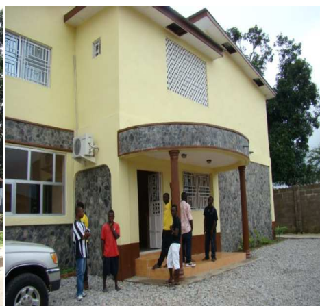
Figure 15 - Rehabilitated Bo Growth Centre
