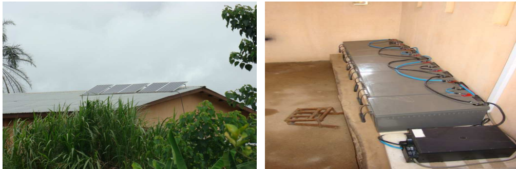
Figure 6 - Small PV system (1 kW with batteries) in Koindu, also at Bo, Pujehun and Kpandebu
