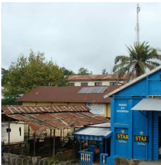
Figure 2 - Existing 1 kW PV system in Bo
