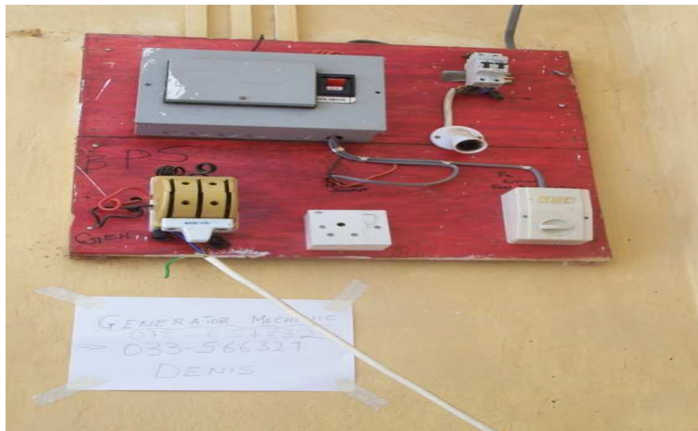
Figure 1 – Solar energy with generator back-up
