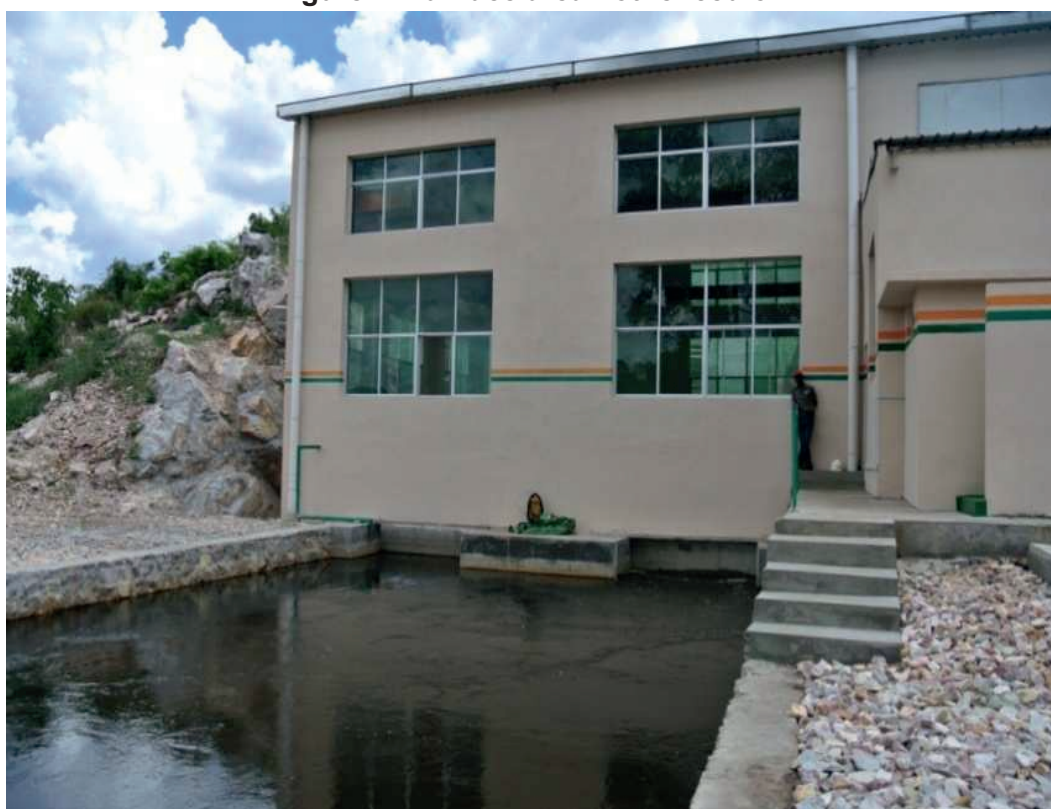
Figure 4: Tailrace area not fenced off
