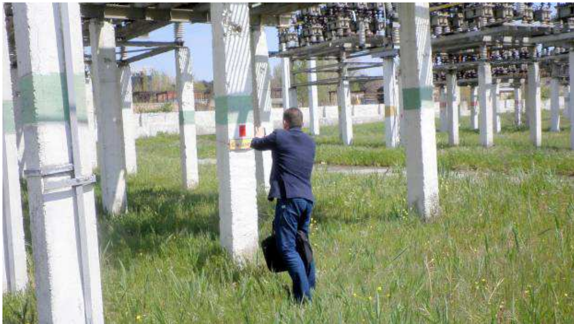
Picture 4. The labelling of the capacitors. When the label is red it means that after the analysis is discovered that the capacitor contains PCB oil. The label is green when it is ascertained after the analysis that the capacitor is free of PCB.
