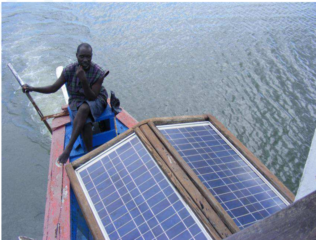
Figure: A small offgrid solar PV system
