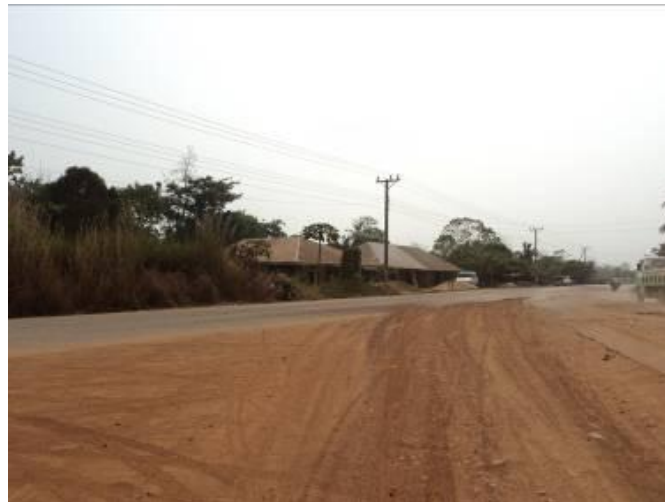
Figure 24: Commercial establishments at a distance of 1 km
