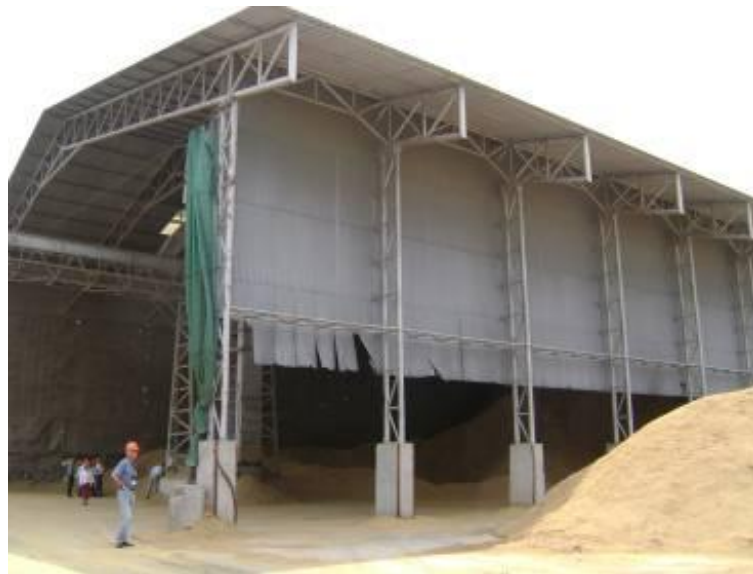
Figure 13: Typical covered shed
