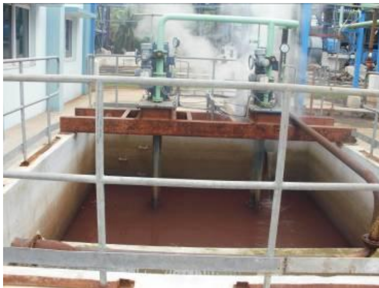
Figure 29: Typical neutralisation pit
