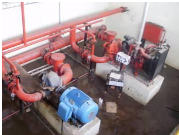
Figure 30: Typical fire fighting system
