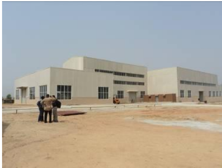
Figure 4: 12 tph rice mill in Ikwo cluster
