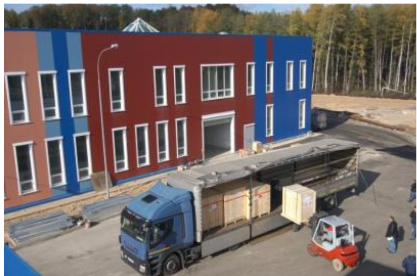
Delivery of equipment to the plant
