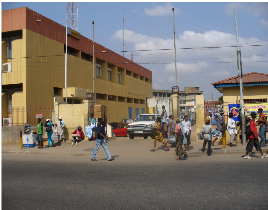
Figure 1.2 The Electricity Company of Ghana's Accra Sub-Transmission Region, Makola, Accra, Ghana
