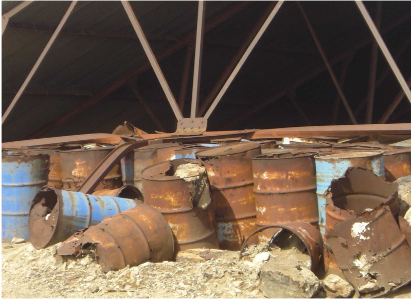
Figure S7 Obsolete pesticides in corroded containers under the collapsed sheds
