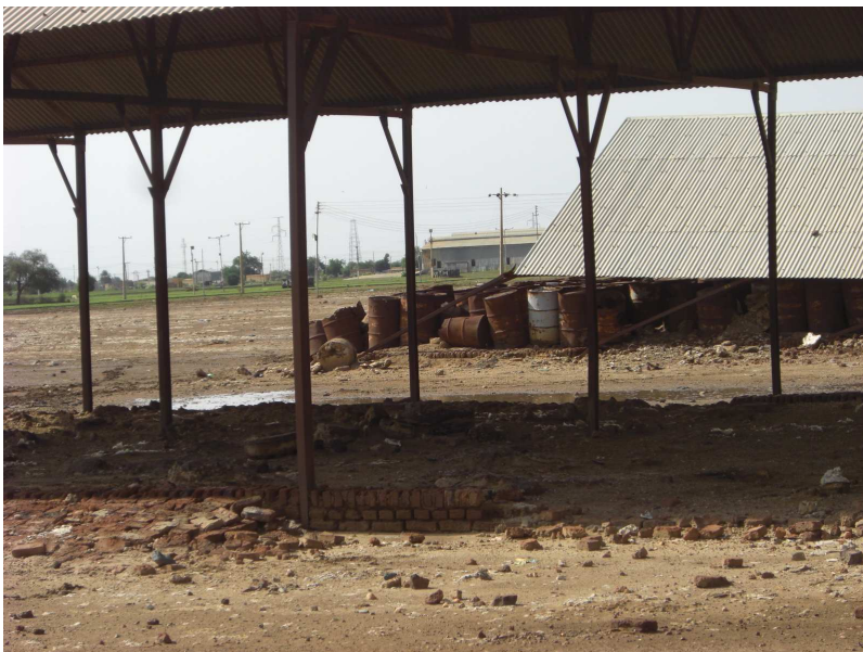
Figure S6 One of the sheds has been cleaned
