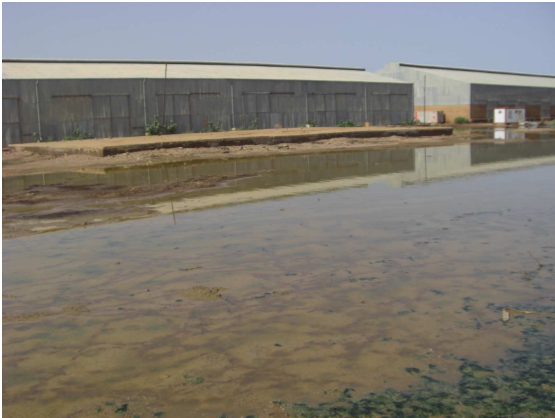
Figure S8 Containment system: the contained dump is still in good condition. Water has no colouring
