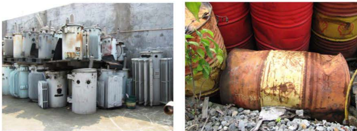
Fig. 4.1.4. Unsafe handling of PCB transformers and PCB oils.
