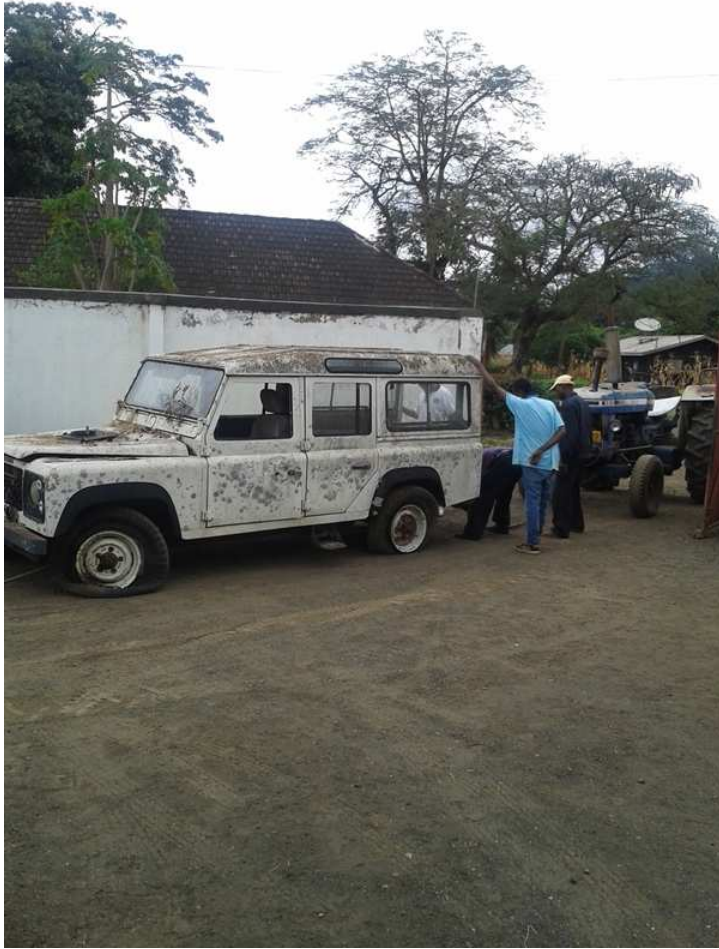
Clearing the site using a tractor
