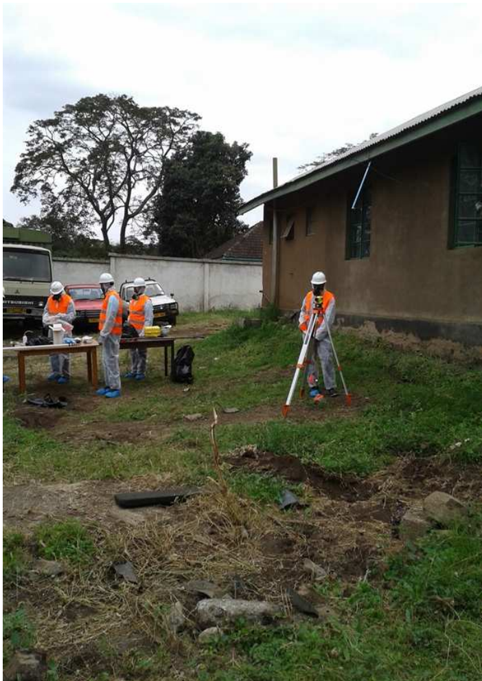
Site survey using topographic Abney level
