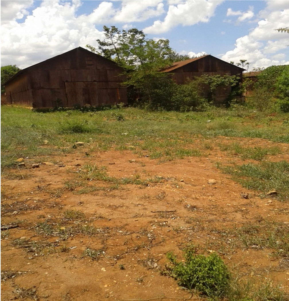
The two storage areas located at the entrance of NHC site in Morogoro- Dec. 11 th , 2013
