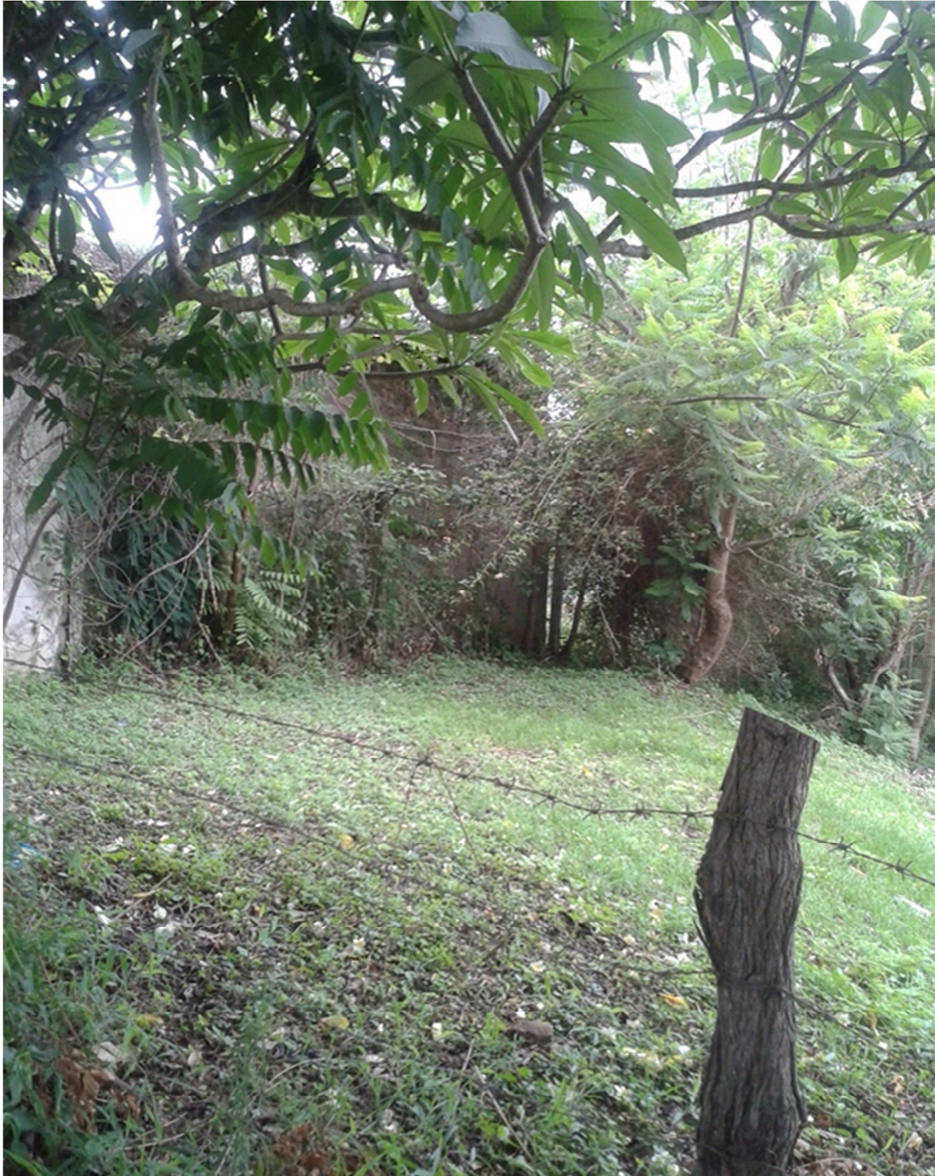
A slope (which is connected to a water stream) lies outside of PPO premise- Dec. 13 th , 2013
