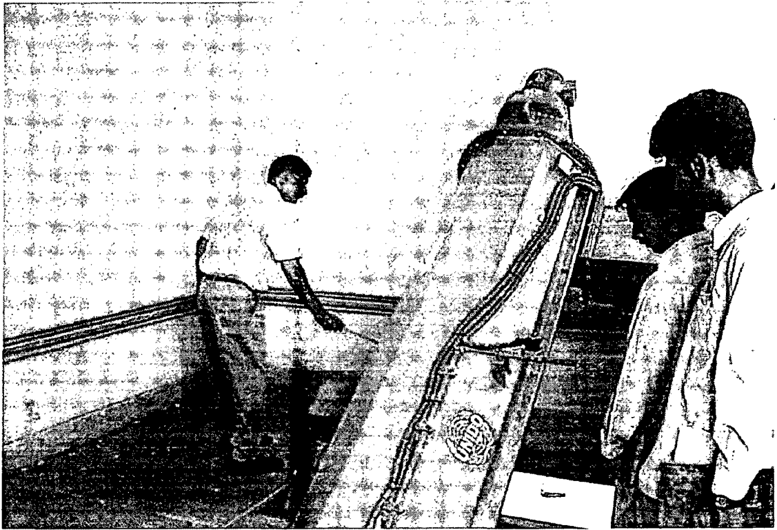
27 - AUTOMATIC SCREEN IN OPERATION
