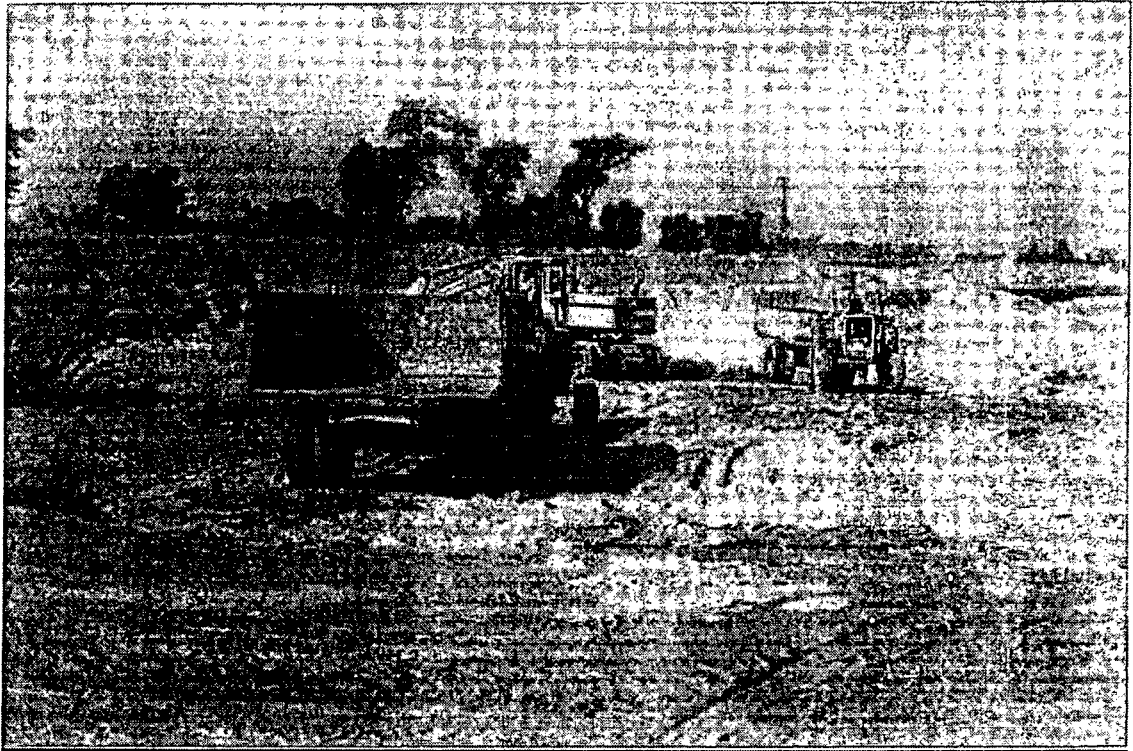
3 - EXCAVATION UNDERWAY FOR LAGOONS
