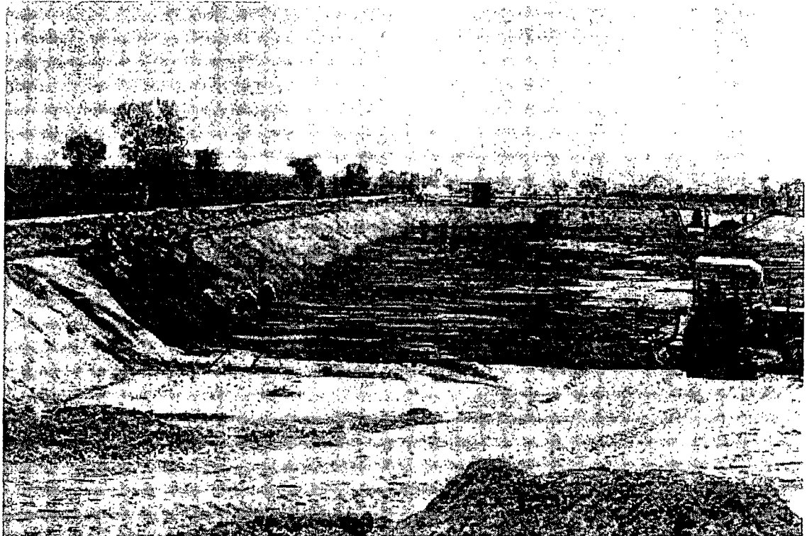
18 - PREPARATION OF DIKES FOR EFFLENT LAGOONS
